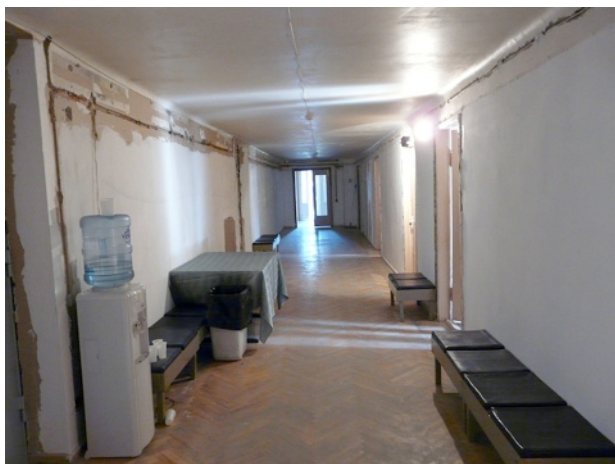
Corridors in Daugavpils Culture Centre, which still need renovation
